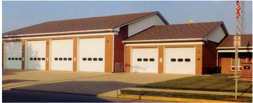
A Rustic Shingle aluminum shake was selected for this fire department in Piqua, Ohio. It boasts reflective coatings, called Hi-R Finish by Classic Products. CLASSIC PRODUCTS PHOTO
