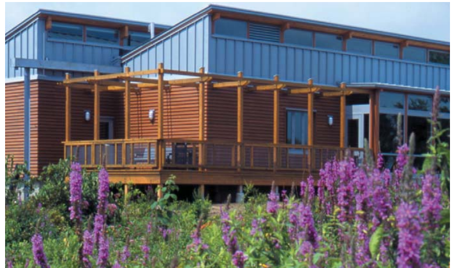
The Parker River Wildlife Refuge in northeast Massachusetts features an Energy Star-compliant standing seam roofing profile from Englert. ENGLERT PHOTO
